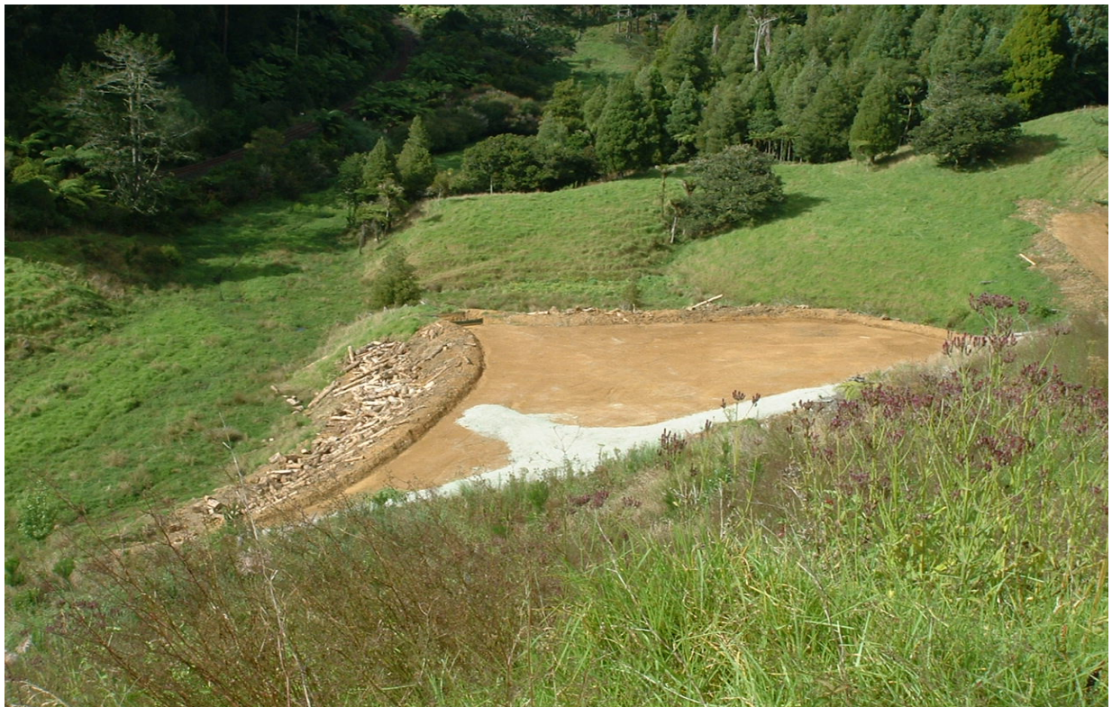
Photo 9.1 Landing Site with bunded edges to direct water flow into decanting earth bund prior to discharge. Slash & offcuts used as stabilisation of embankments. Decanting earth bund located at upper point of landing. Landing area less than 3,000m 2 .
