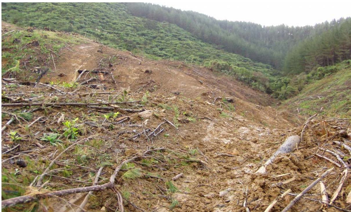
Photo 9.4 A practice to be avoided. Blind hauling 'sweeping' sediment into watercourses as well as unnecessarily exposing earth.
